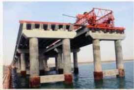
BOUBYAN ISLAND SEAPORT PROJECT (PHASE 1, STAGE 1), KUWAIT Bridge part includes a 1.42km road bridge and a 4.25km railway bridge across Subiya Straits 2011 Supply of post-tensioning system
