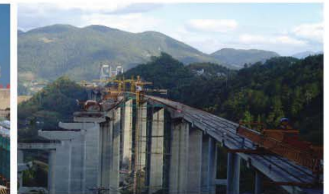
SHUINAN GRAND BRIDGE AT HURONGXI HIGHWAY, CHINA Left bridge 917.75m, right bridge 953.23m, highest pier 98m 2008 Supply and installation of PT
