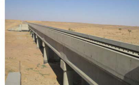
North-south Railway, KSA 2011 Supply of anchorage, bearings and expansion joints
