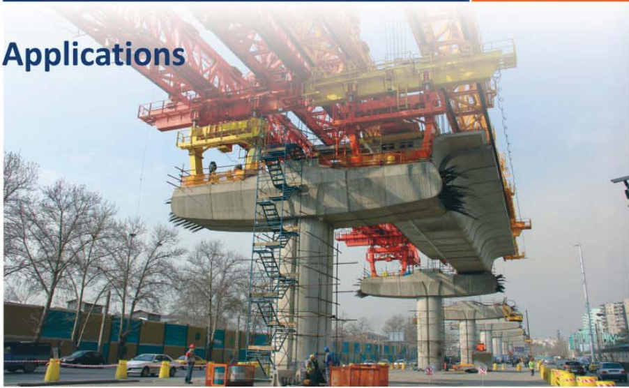
Sadr Bridge, Iran, 2012
